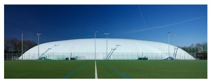
Hockey hall 6,400 sqm - "supported and heated" by 2 units type K300/D (total air output 48,000 cbm/h)
