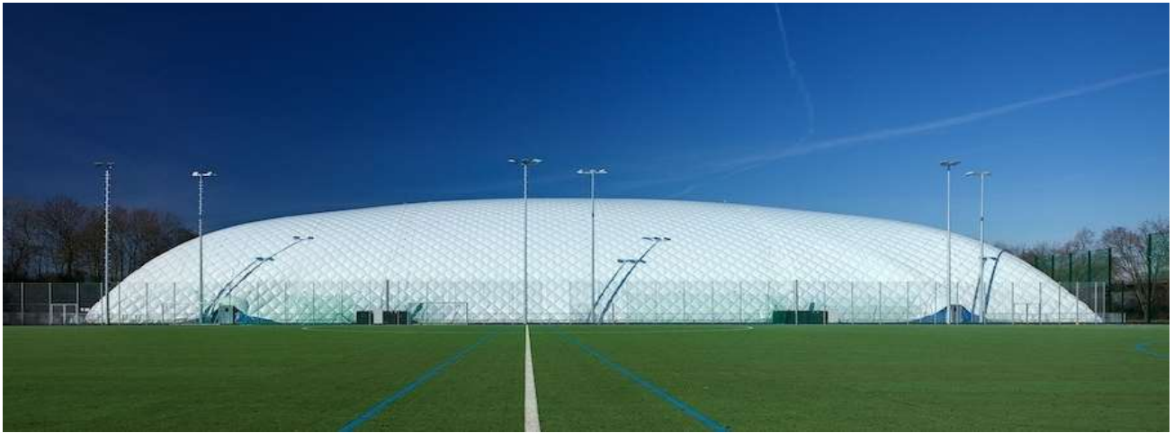
Hockey hall 6,400 sqm - "supported and heated" by 2 units type K300/D (total air output 48,000 cbm/h)
